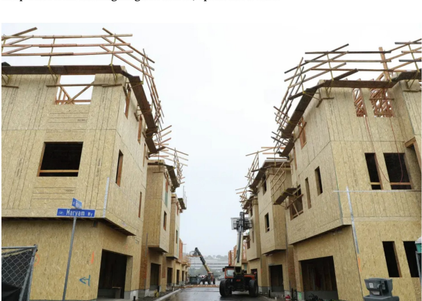
New construction at City Village being built by SummerHill in Bishop Ranch. Les Suzuki/S.F. Chronicle
